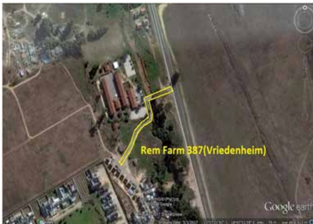
Fig 3: Possible access route
